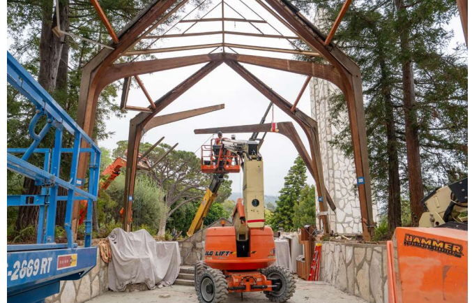
Disassembly of the structural redwood bents.
