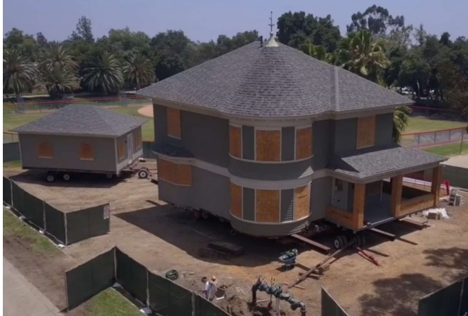
Renwick House at its new location, prior to construction of a permanent foundation.
