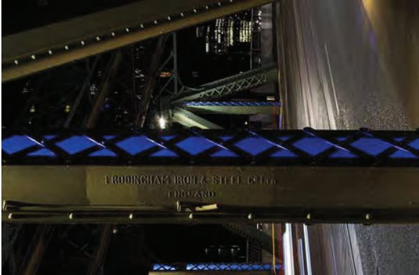
STRUCTURAL METAL BRACING WITH RIVETS
