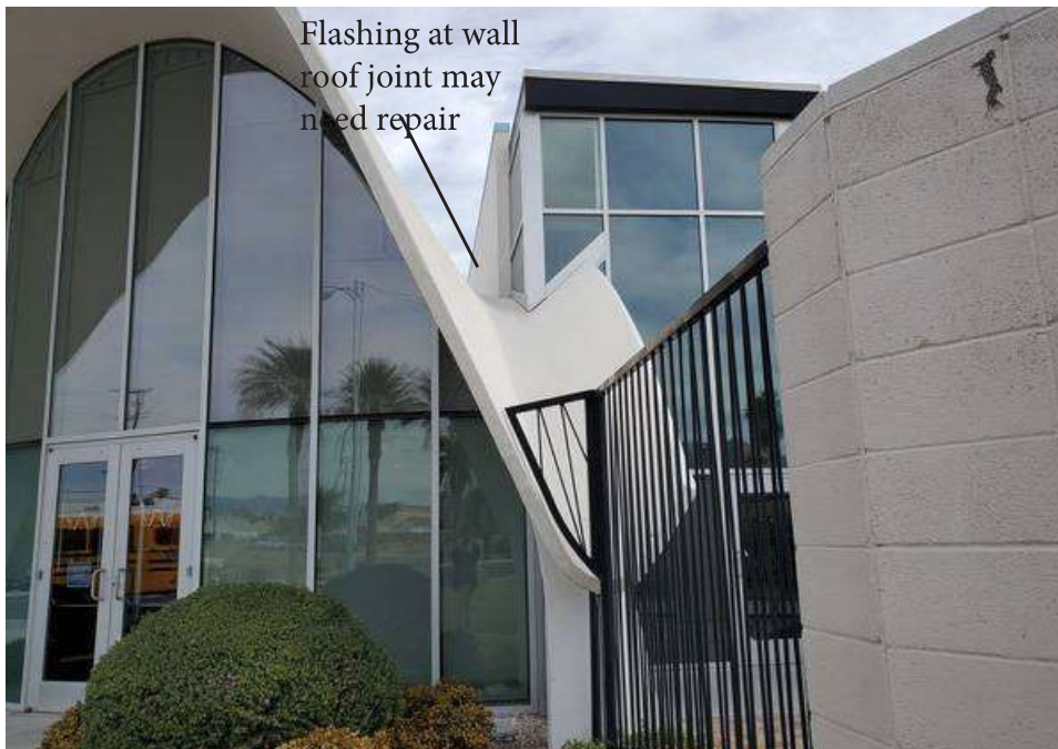
Photo 6 - The shell and vertical wall intersection needs to be flashed to properly direct the water. Possible water intrusion may occur along the roof in the areas shown and at the window. This needs to be inspected and repaired.
