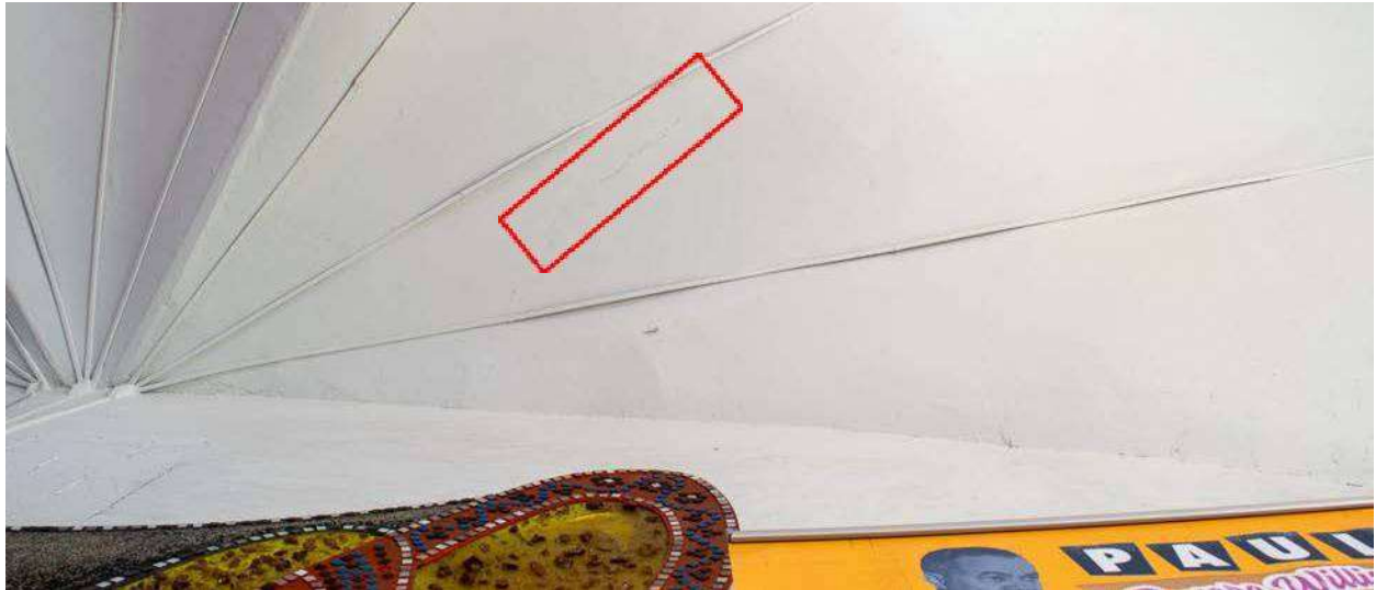
Visitor Center Soffit: Visible crack, approximately 18" in overall length, close to the back wall
