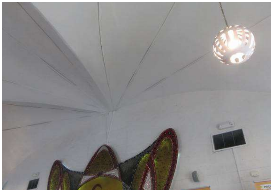
Photo 3 - Interior wiring today. In many areas the wires have lost their adhesion to the ceiling plaster.
