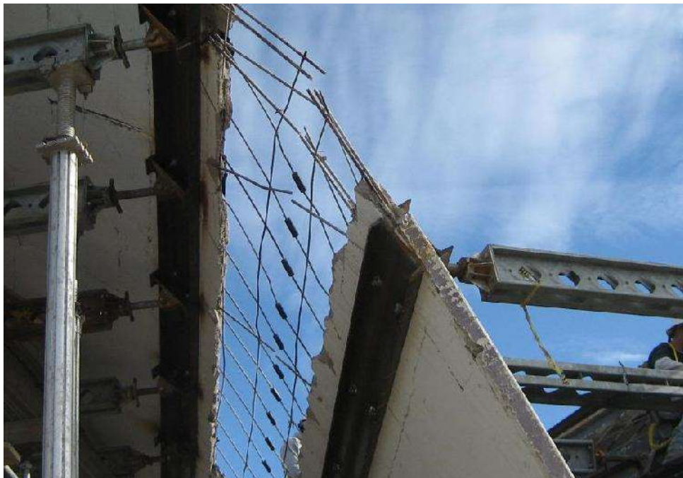
Photo 5 - Example of the joint between the several concrete sections. Mechanical splices can be seen. In some cases, because of the reinforcing steel was too close to the surface, welding was required.
