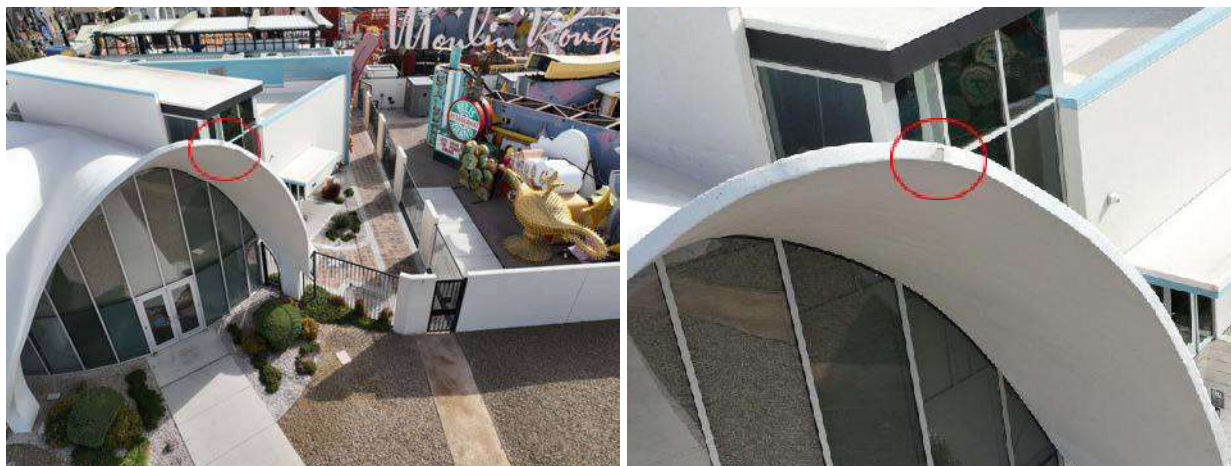
Membrane Damage: Image of defective membrane at north west roof overhang
