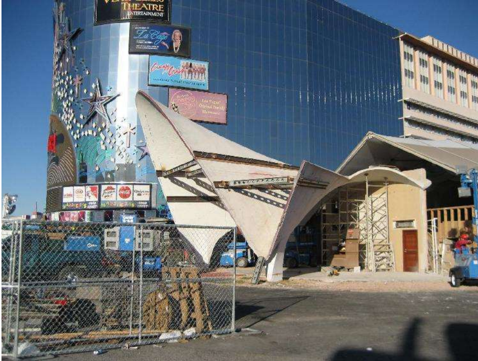
Photo 4 - This photo shows how the various sections of the shell were cut. The sections were then stored for reassembly.
