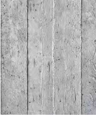
BOARD-FORMED CONCRETE
