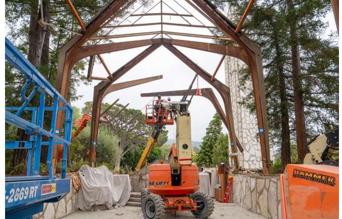
Disassembly of the structural redwood bents.
