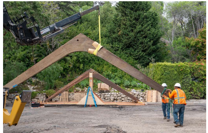
Structural wood members are stored in custom-designed cradles.
