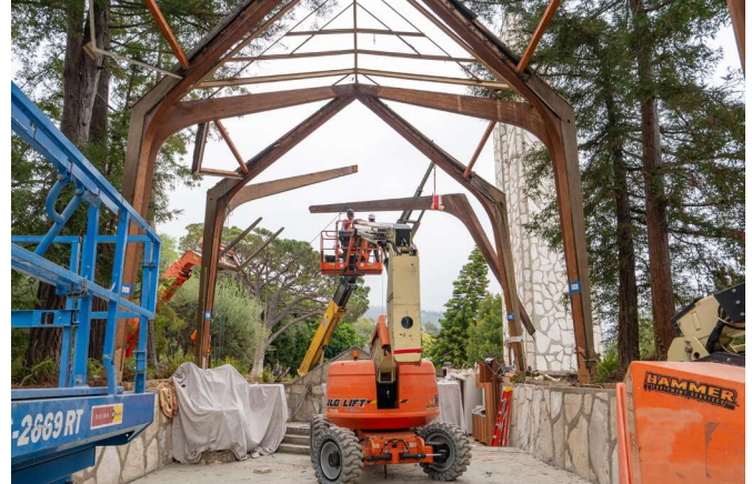
Disassembly of the structural redwood bents.
